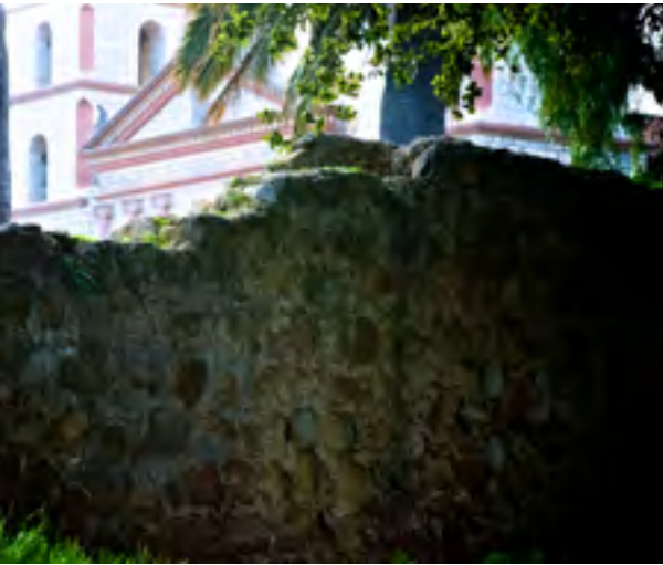
Figure 5-31, Right: Ruins of upper reservoir. The remains of an aqueduct feeding this reservoir can be seen in the foreground. Built in 1827 to store water for the grist mill, the penstock (circular hole at base of wall) was fitted with a wooden gate that controlled the flow of water which turned the wheel of the mill's grindstones.
