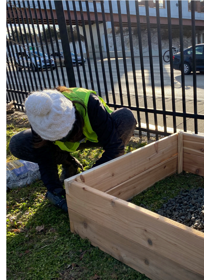
↑ Image: Installation of soil plots
