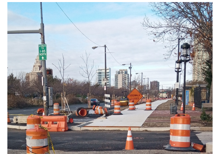
↑ Image: Pre-installation. view from the intersection.
