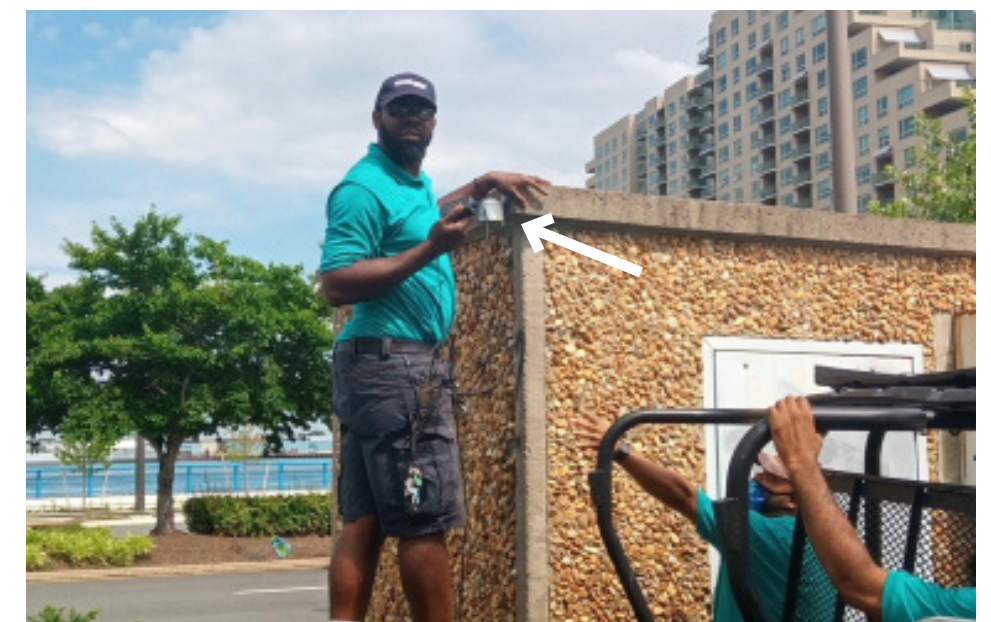
Image → Installation of PurpleAir at the I-95 site.
