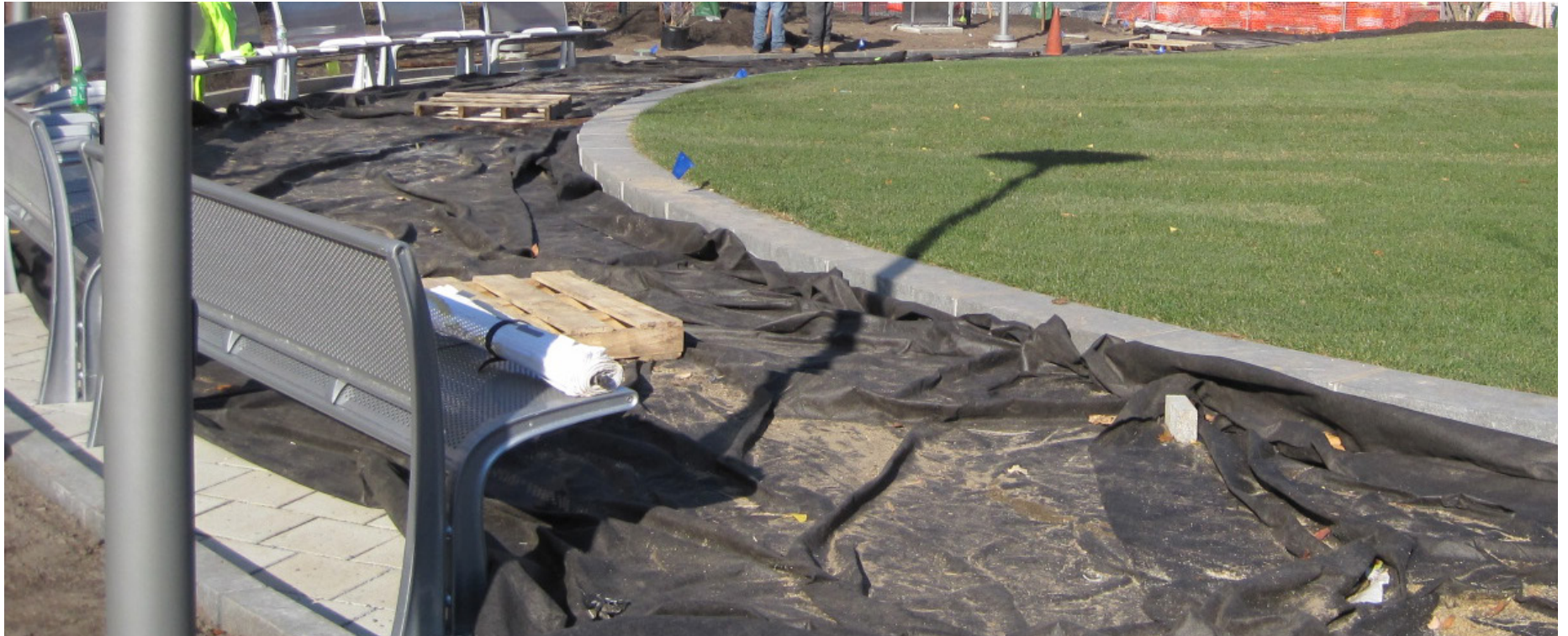
Kane Park Geotextile Installation, Credit MNLA
