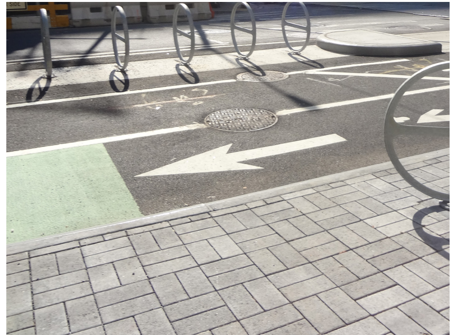
Figure 5.04, Permeable Paver at Streetscape, Credit MNLA
