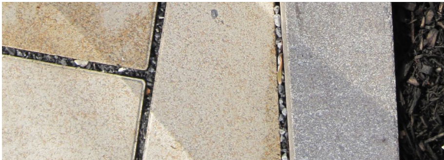
Figure 5.02, Permeable Paver Joints, Credit MNLA
